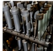
Capacitor Bank Replacement & kVAR Upgrading
