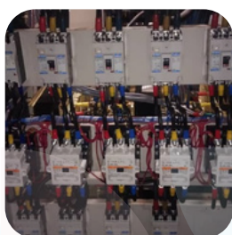
Replacement of Contactor
