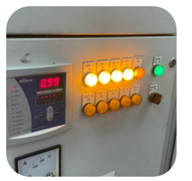
Result: PF increase to optimum level @0.99
