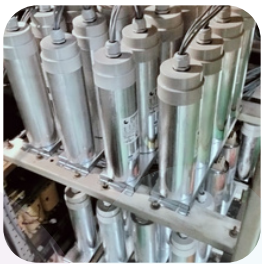
Replacement Upgrading Capasitor Bank
