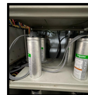
Replacement Parts & Components of Existing Capacitor Bank
