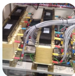
Replacement of Reactor
