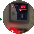
Power factor unit at incoming distribution
