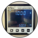
Power factor unit at inverter
