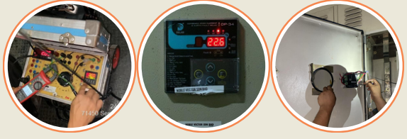
Protection Relay Installation and Calibration
