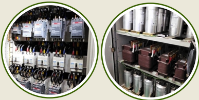
Capacitor & Reactor Replacement/Upgrading
