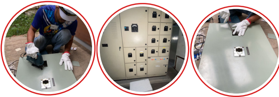
Panel Fabricating & Protection Relay Installation
